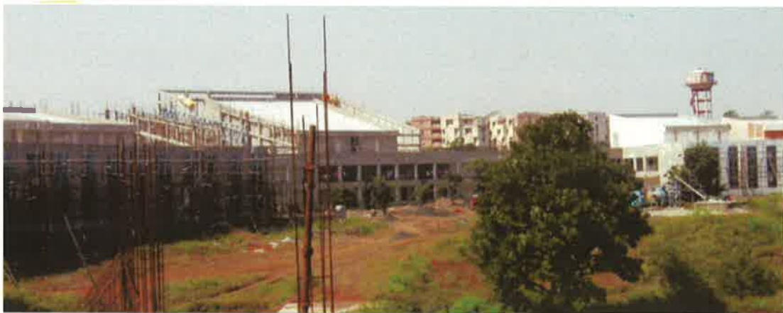
Lecture Hall and Tutorial Complex under construction
