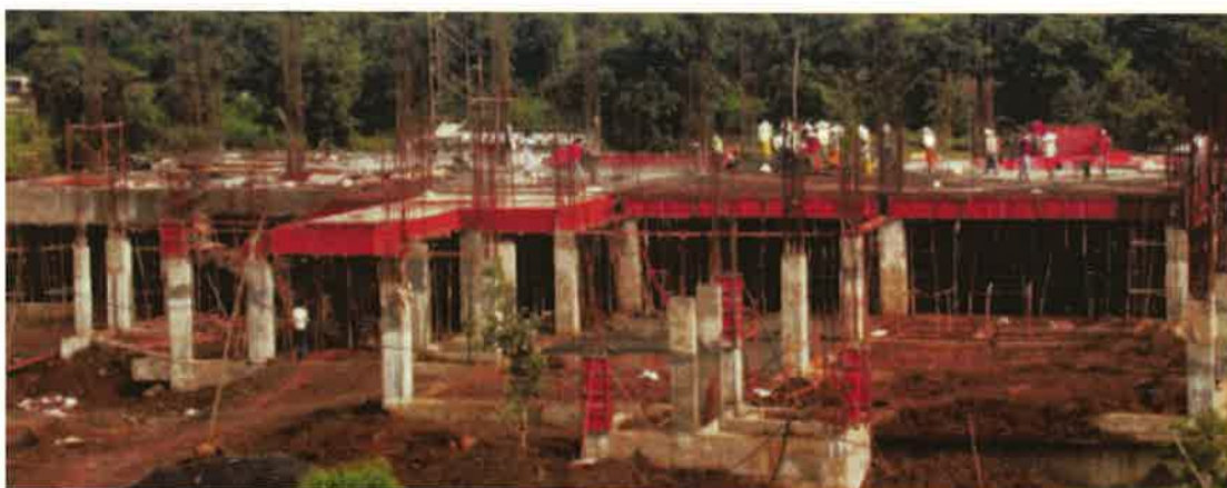
Library-cum-Computer center under construction
