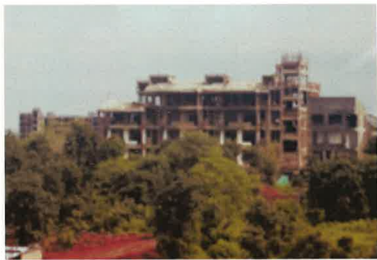
Visitors Hostel under construction
